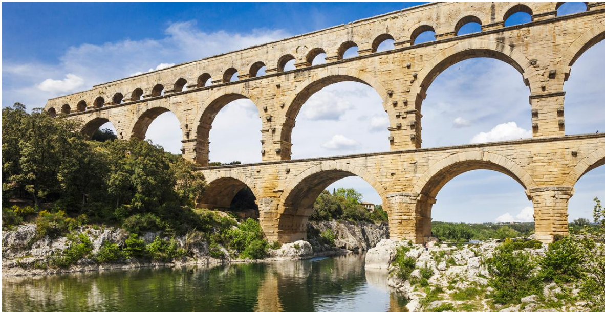
Bridge of the Gard (F)...
